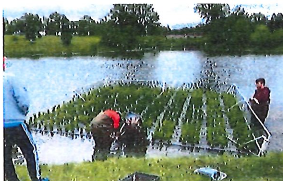
Figure 4. UNL Students assembling a floating treatment wetland at Cooper YMCA in Lincoln NE
