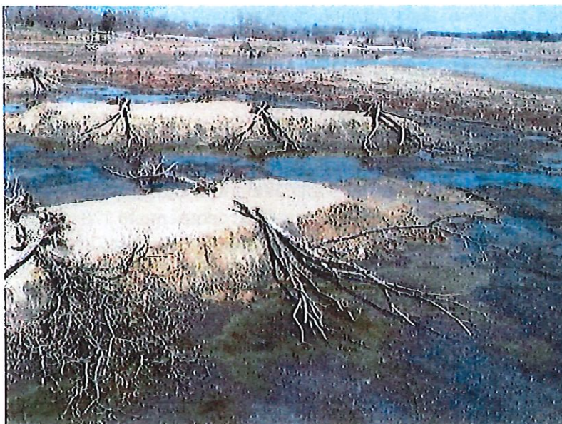
Figure 9. Log Crib / Root Pile. Underwater "islands" were left in place as sediment was removed from around them. The photo also shows trees anchored with weights and cables to provide fish habitat features (photo above from Conestoga Reservoir during lake drawdown).
