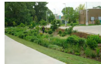
BIOSWALES/RETENTION OR INFILTRATION BASIN
